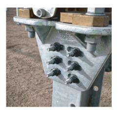
Recent research done by a national energy company during a routine ten-year inspection at a solar farm found zero failures among thousands and thousands of Huck fasteners they used. Other fasteners in the same location had issues of fatigue breakage, corrosion and loss of clamp force. The HuckBolts used on racking systems did not require a single day of maintenance.
